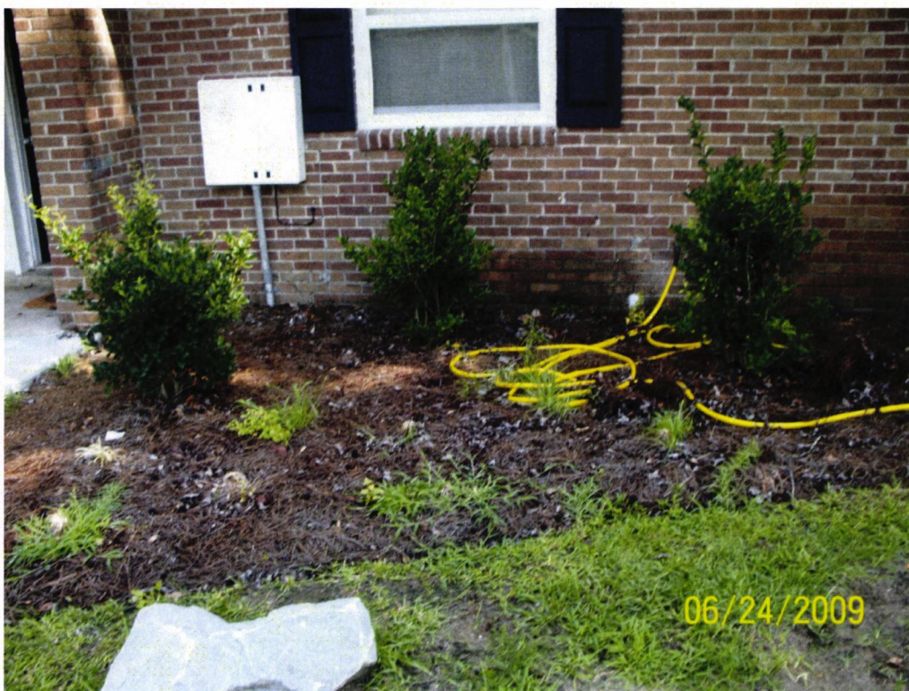
Picture 1: Location of UST 1161Jasmine prior to excavation.
